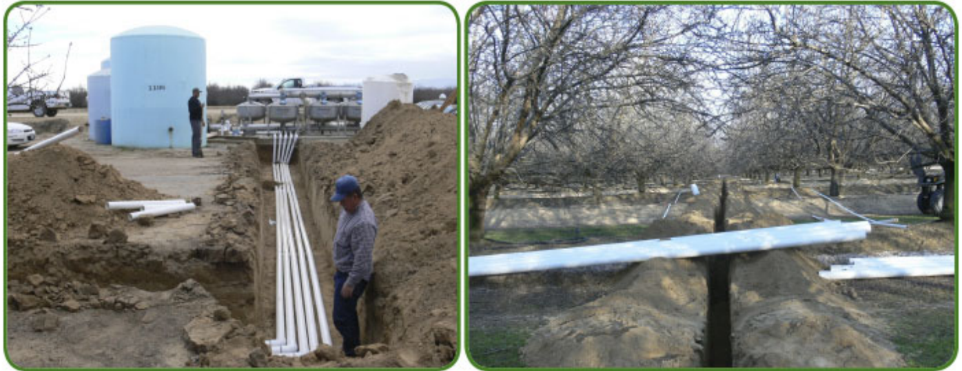
Figure 2a y 2b. Preparing the orchard for irrigation, with double line drip (8 emitters per tree) or fan jet sprinklers with an 8 foot diameter throw (2 per tree). All treatments received 48-52 inches of irrigation scheduled according to evapotranspiration measured on site.
